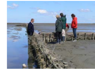
Brushwood dams contain the silt deposits
